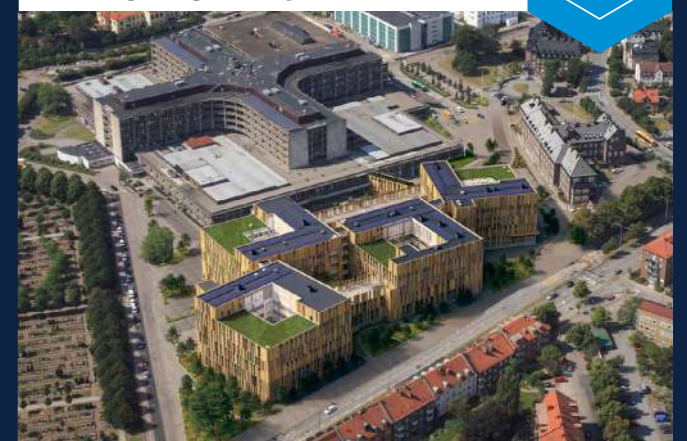
REGION: SCANDINAVIA Helsingborgs Hospital
